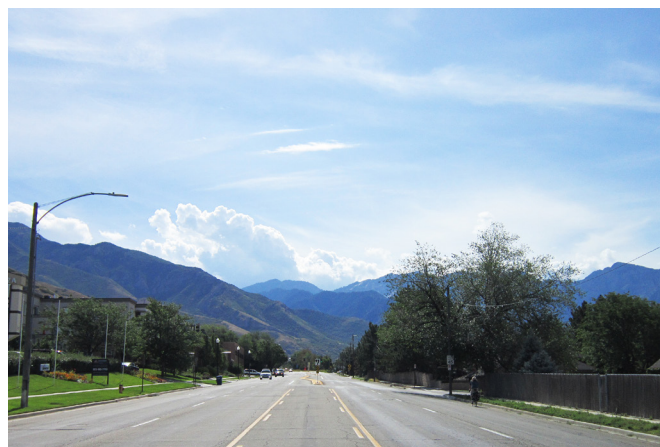
A view of a current typical cross section of the Parley's Way corridor, with a center turn lane and no raised median.
