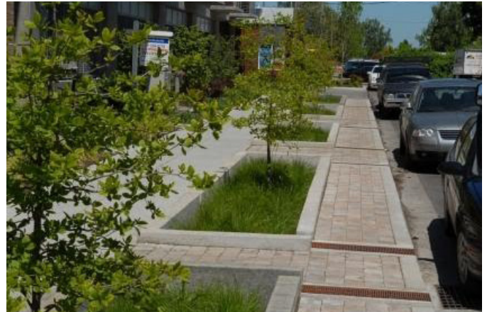
Sidewalk plantings are designed to improve storm water runoff and to create a desirable pedestrian experience
