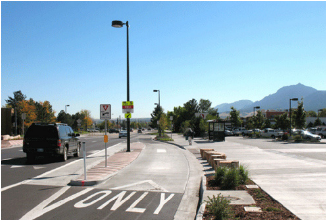
Bus pullouts allow for efficient traffic flow, shared lane with bicyclists, convenient loading and safe pedestrian crossings
